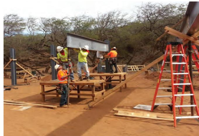
*Hakioawa's remote location and the inability to bring heavy machinery to the worksite forced our build team to rely on manpower to erect and complete the Hakioawa Hale Project.*
